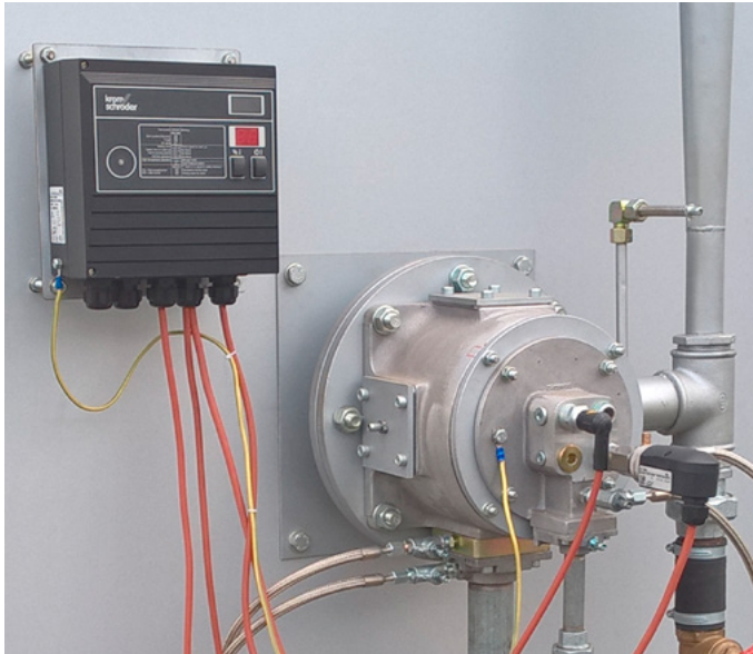
ECOMAX burners with burner control unit BCU
