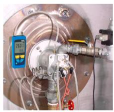
A magnet on the reverse side of the device allows hands-free operation, e.g. during adjustment work on the burner.
